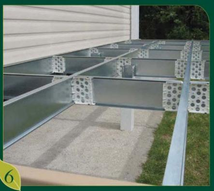
The steel sub-frame is simplicity itself. It consists of just two components - a steel T beam and its connector. The sub-frame is easily connected into a grid pattern and the deck boards are fixed directly to the steel joists.
